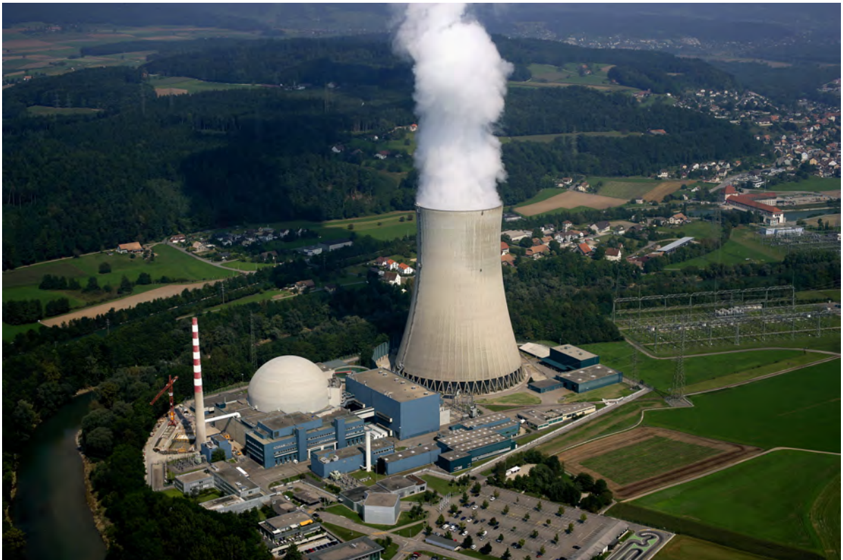
Figure 5-1: Aerial view of the Gösgen nuclear power plant (KKG). Source: KKG
