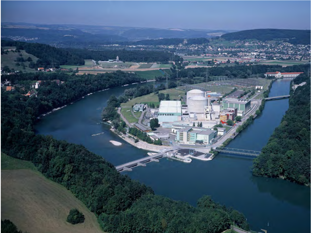
Figure 3-2: Aerial view of the Beznau nuclear power plant (KKB), comprising two units. Source: KKB
