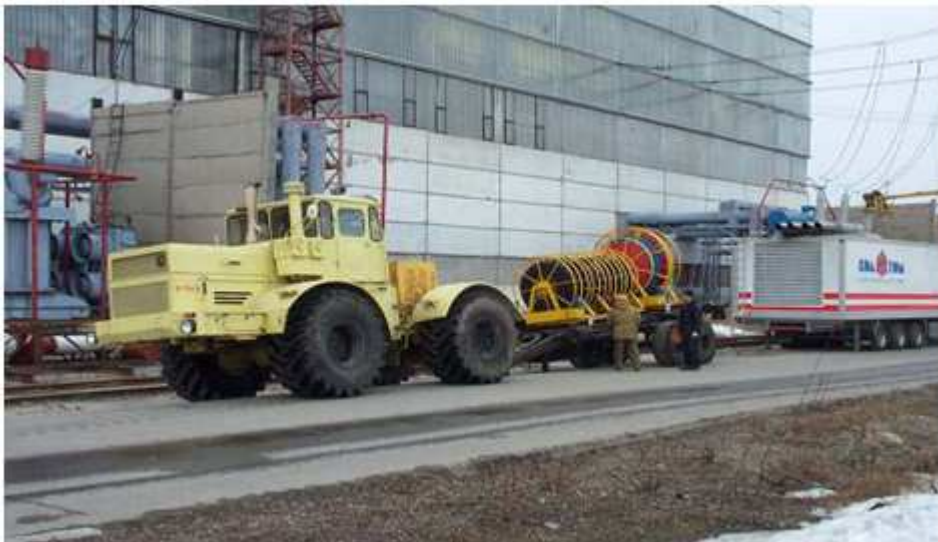
Fig. 2.1. Mobile emergency diesel-generator station, Kola NPP
