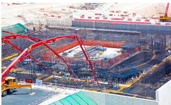
FIG. 1. Construction at Barakah-1 in the UAE (photograph courtesy of ENEC).
