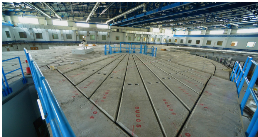
8 To ensure safety, the specially designed roof shield provides radiation protection and protects the storage rings through which the electromagnetic beamlines circulate.
