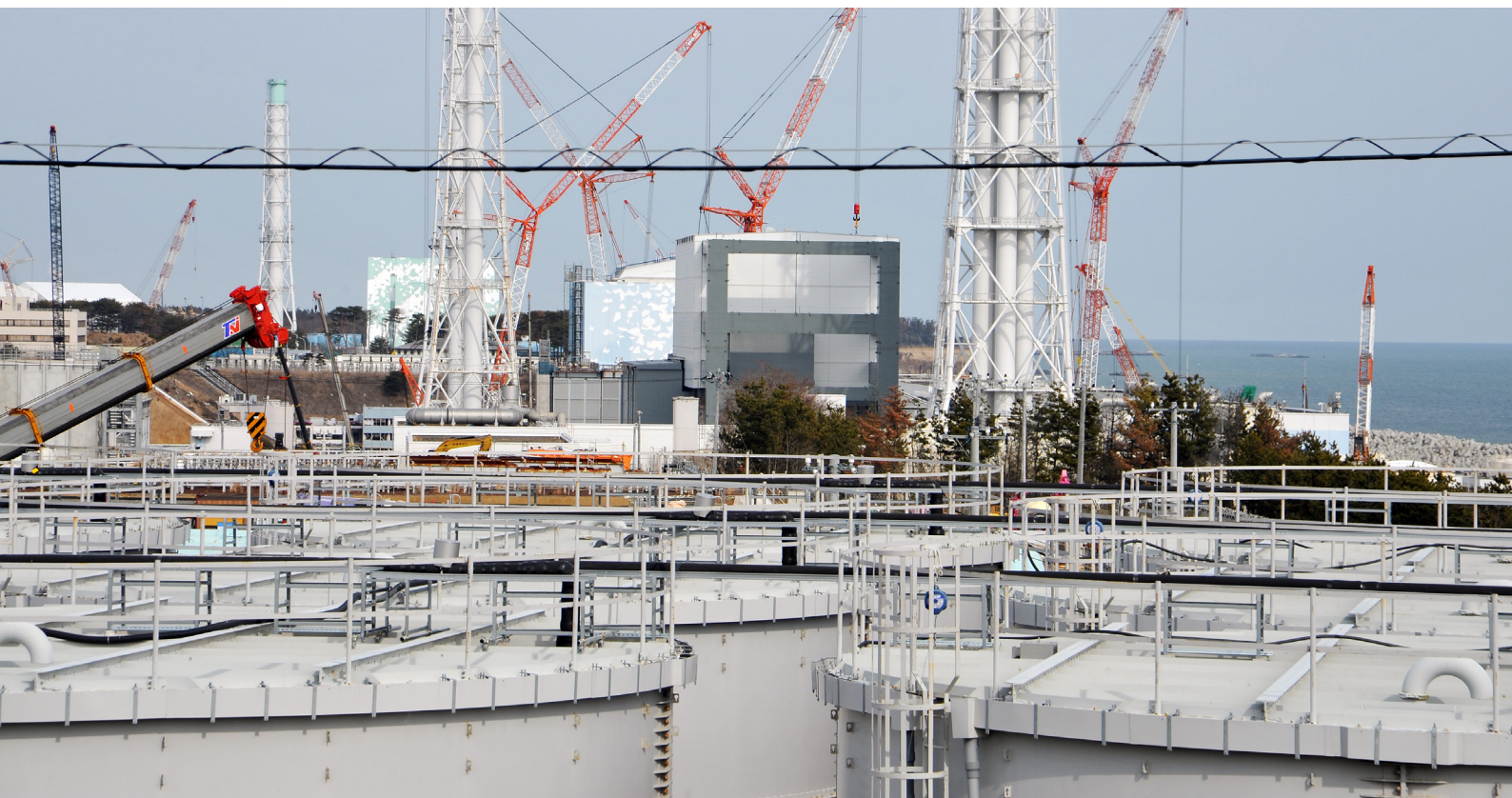
Water tanks holding contaminated water in front of the reactor buildings at Fukushima Daiichi.
