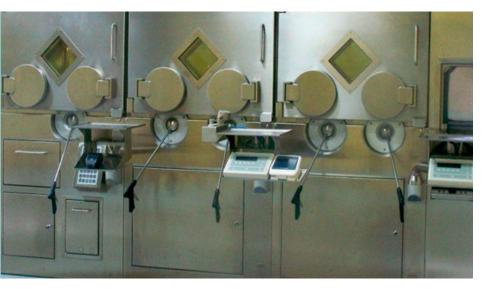
The newly established facility for producing Y-90-based radiopharmaceuticals has good manufacturing practices compliant hot cells for protecting workers and ensuring the production of high-quality drugs.
