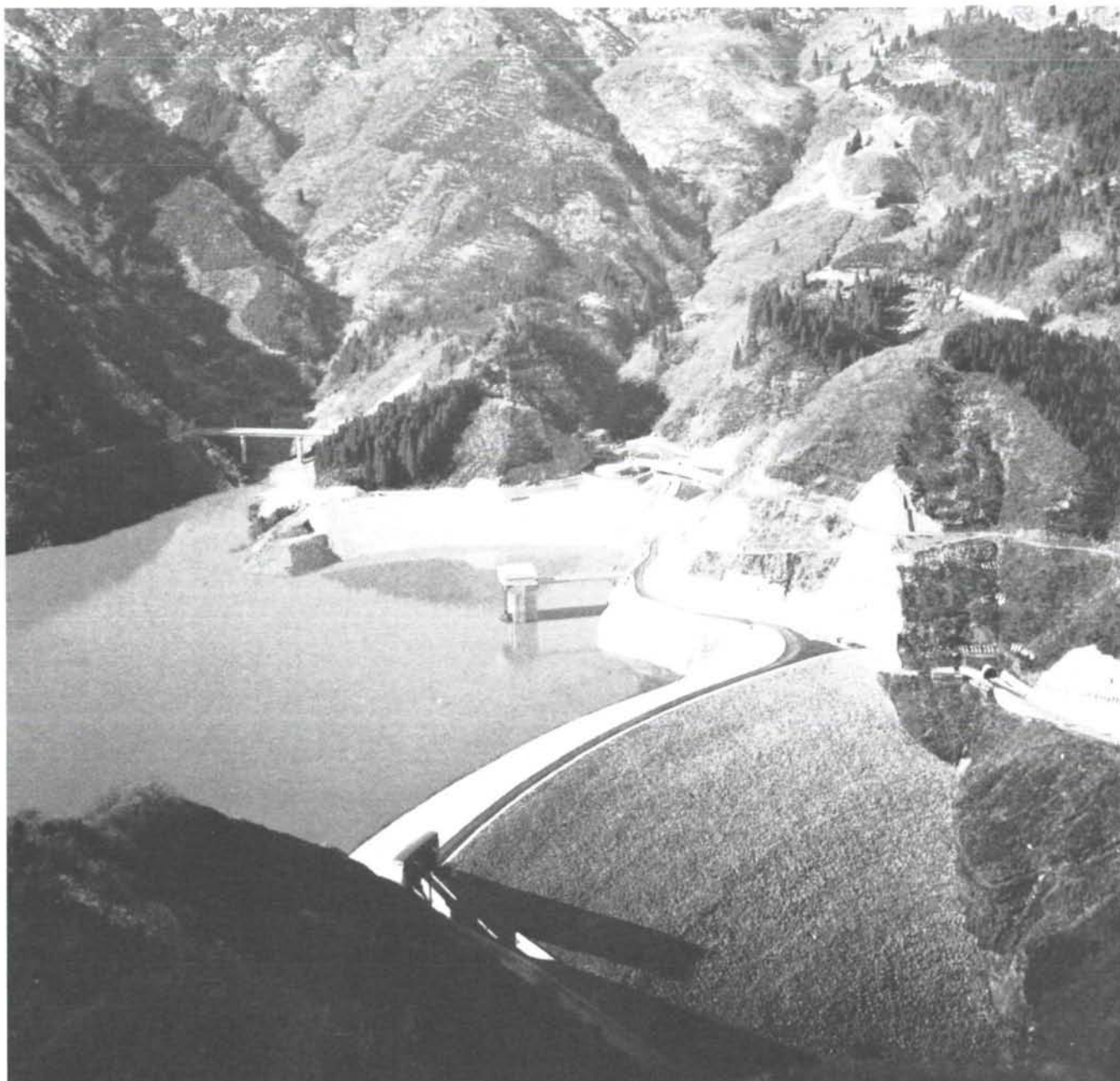
In Japan, nuclear energy and hydropower are major producers of electricity. Shown is the Tedorigawa Daiichi hydropower station. (Credit: JAERI)
