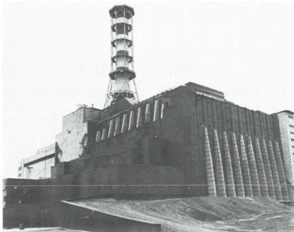
The damaged Chernobyl reactor has been encapsulated in a structure called an "envelope" (generally referred to as the "sarcophagus"), which is intended to contain radioactive materials and prevent environmental contamination.
