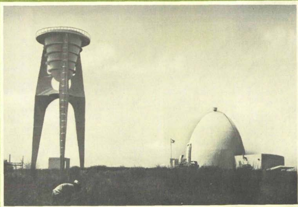
The Philippine Atomic Research Centre at Diliman, Quezon City, showing the water storage tank (left) and the reactor building (right).
