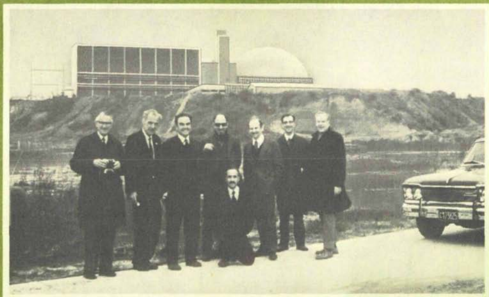
The Puerto Nuevo Steam Plant, Buenos Aires, Argentina, visited by the Survey team.
