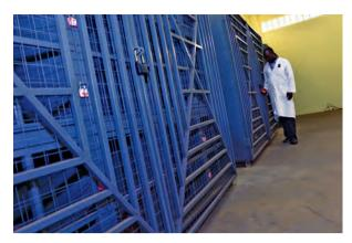
FIG. 2. Secure storage at a facility in Ghana incorporating various types of physical barrier to prevent theft of and unauthorized access to radioactive material.
