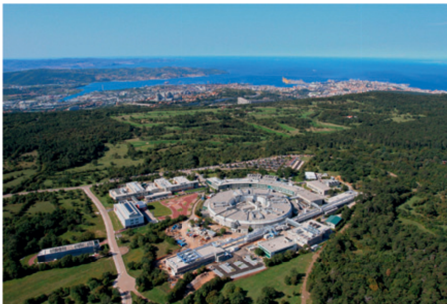
FIG. 3. Aerial view of the Elettra facility, Trieste, Italy.
