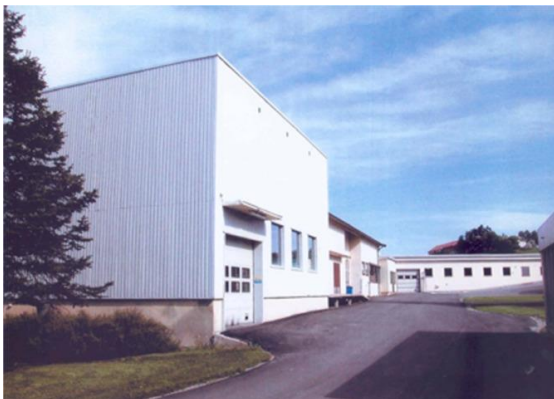
Figure D-4: Radioactive waste facility, Kjeller site
