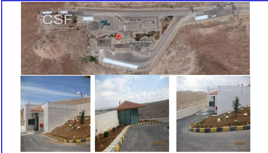
Figure L.1 Central RW Storage Facility at JAEC
