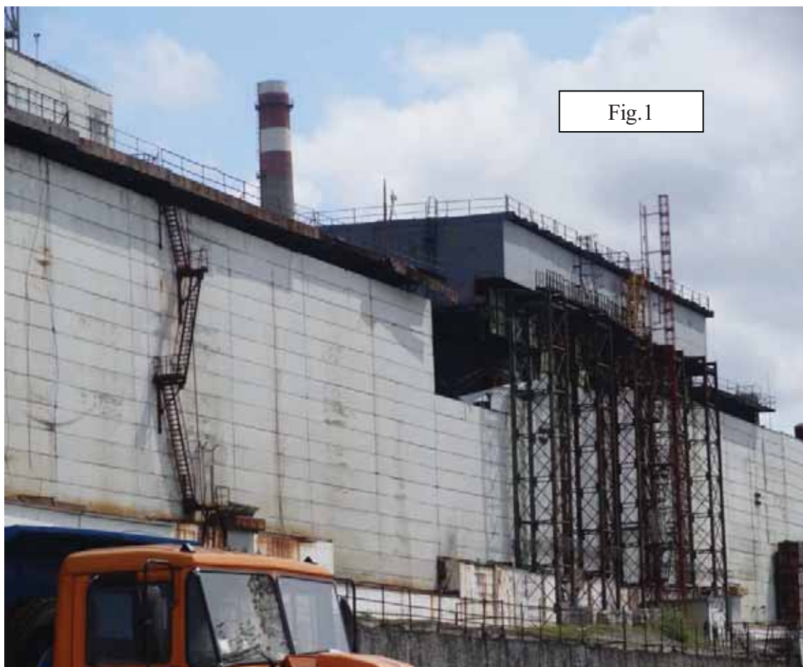
Figure 1 Turbine Building outside view of area of collapsed wall and roof section
