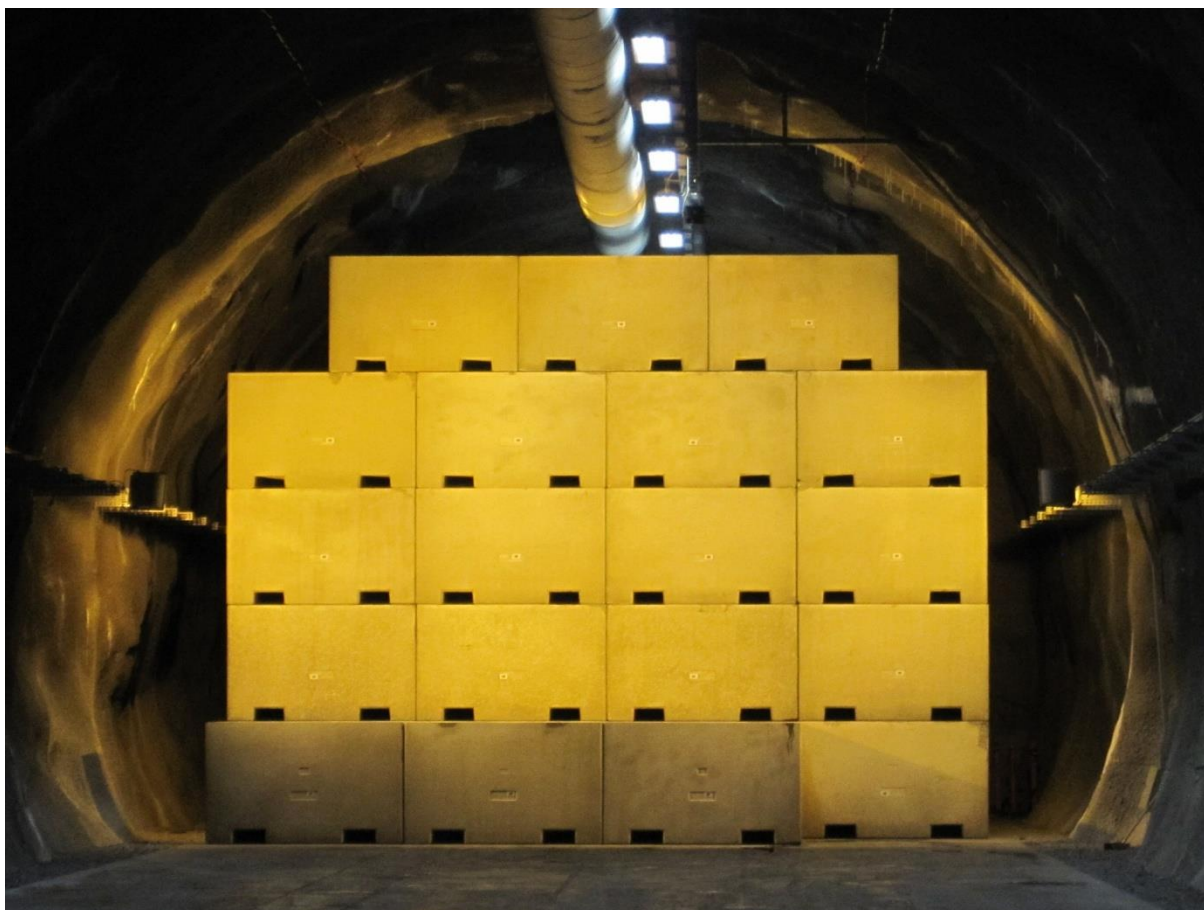
Figure B.2.1 – 3. Containers disposed in the I-K1 chamber of the National Radioactive Waste Repository
