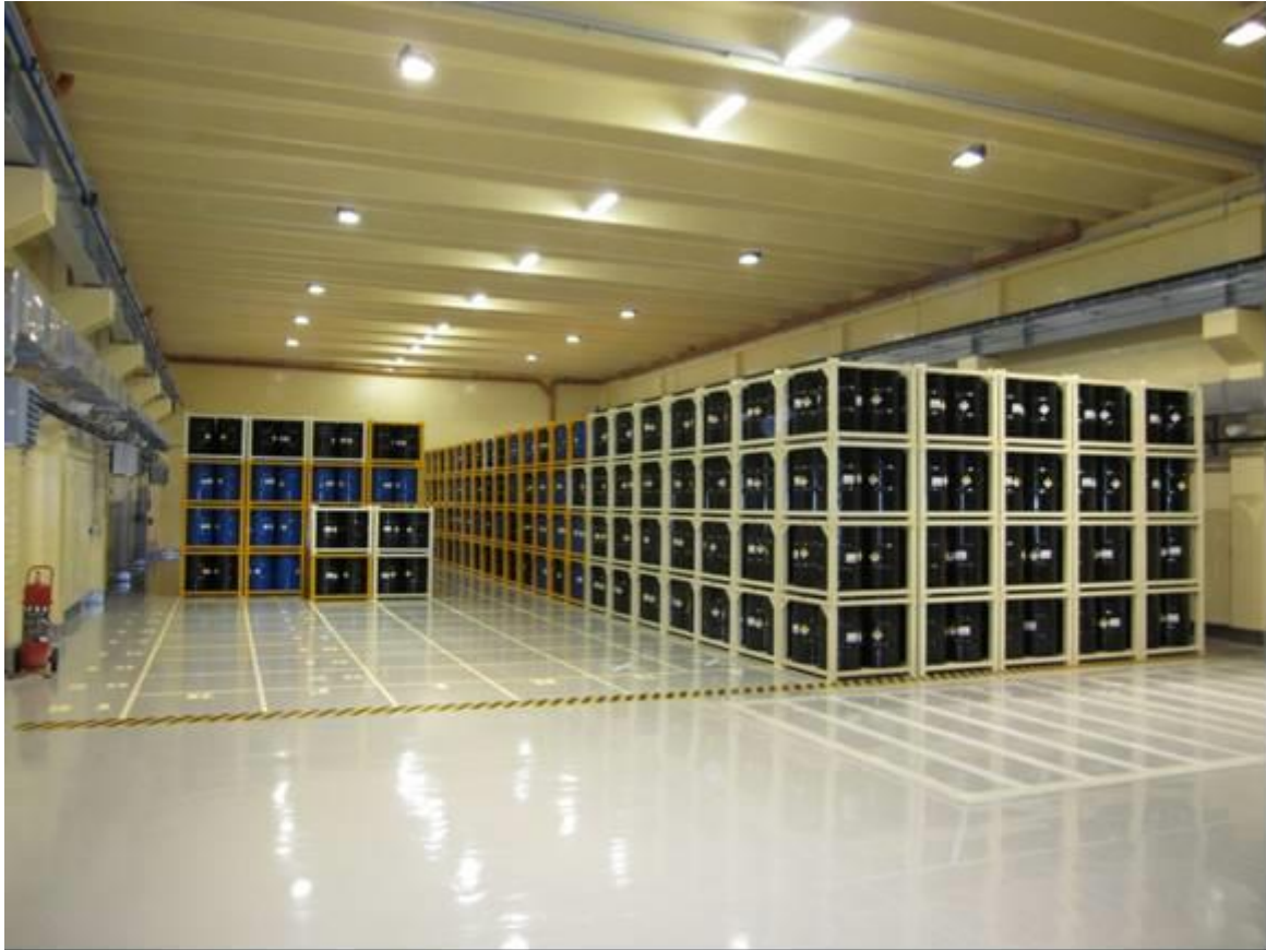
Figure H.3-1 Technology hall of the National Radioactive Waste Repository
