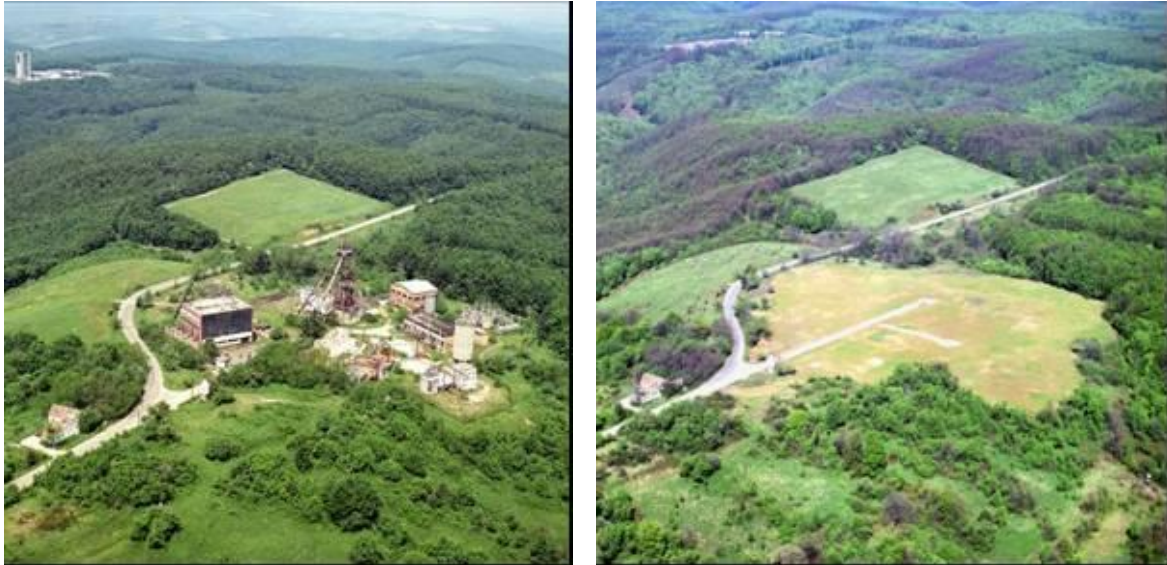
Figure An7.2.4-1: Air shaft IV of the uranium ore mine during operation and after remediation
