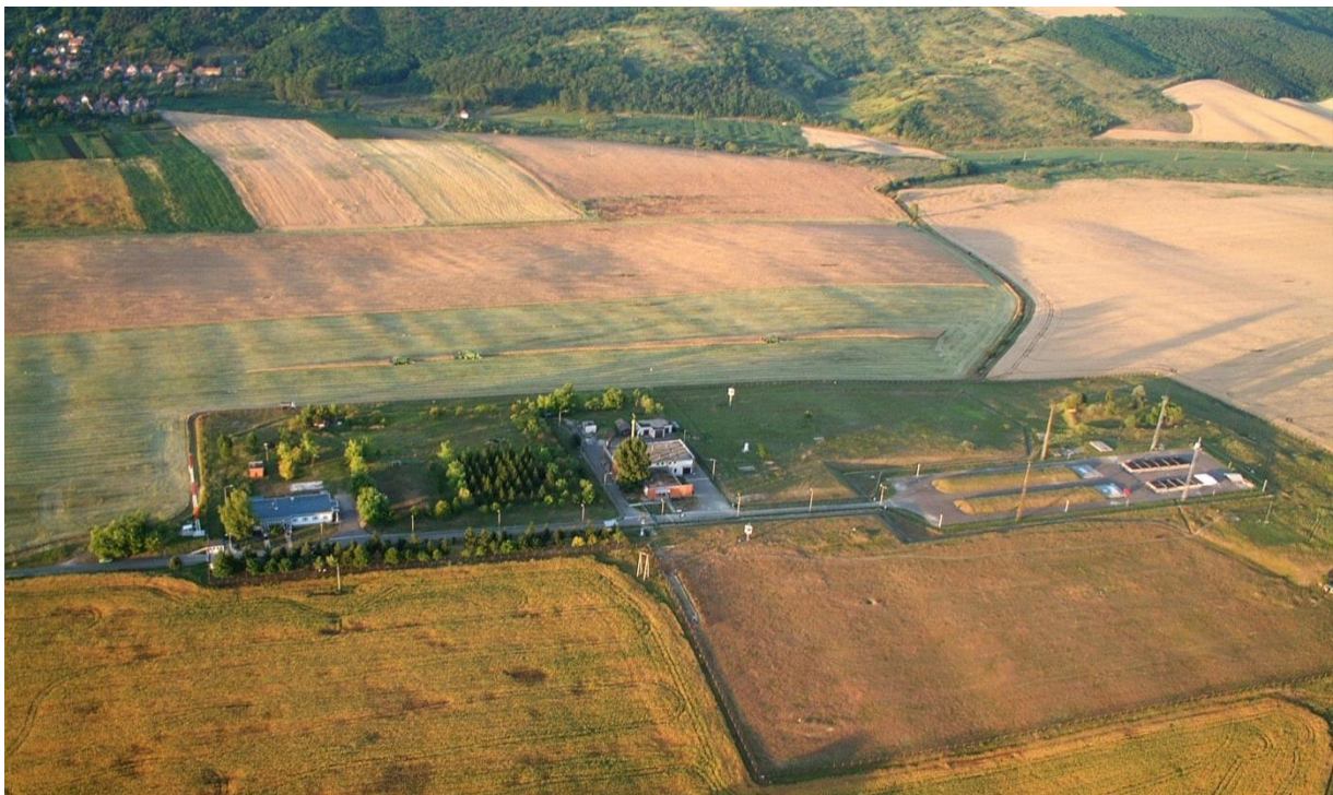
Figure B.2.1-2 Bird’s eye view of the Radioactive Waste Treatment and Disposal Facility
