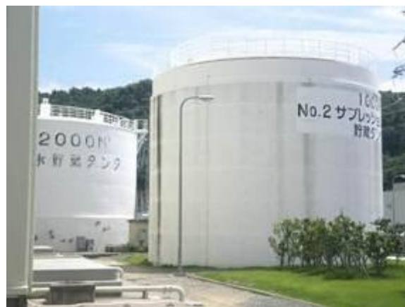
Figure 7-4 Condensate Storage Tank (left) and #2 Suppression Pool Water Storage Tank (right)
