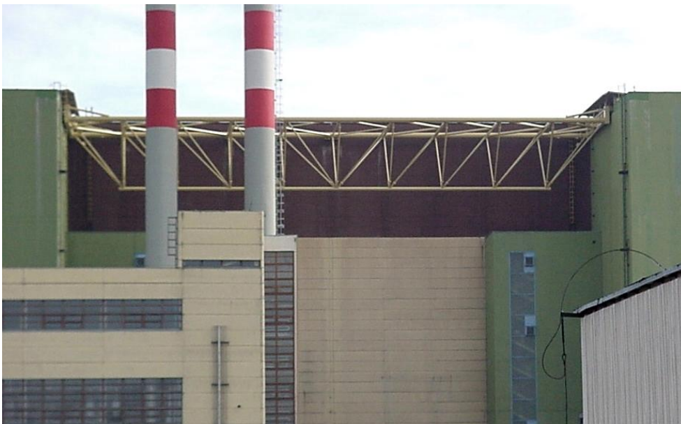
Figure 2-5: One of the reinforcements of the main service building
