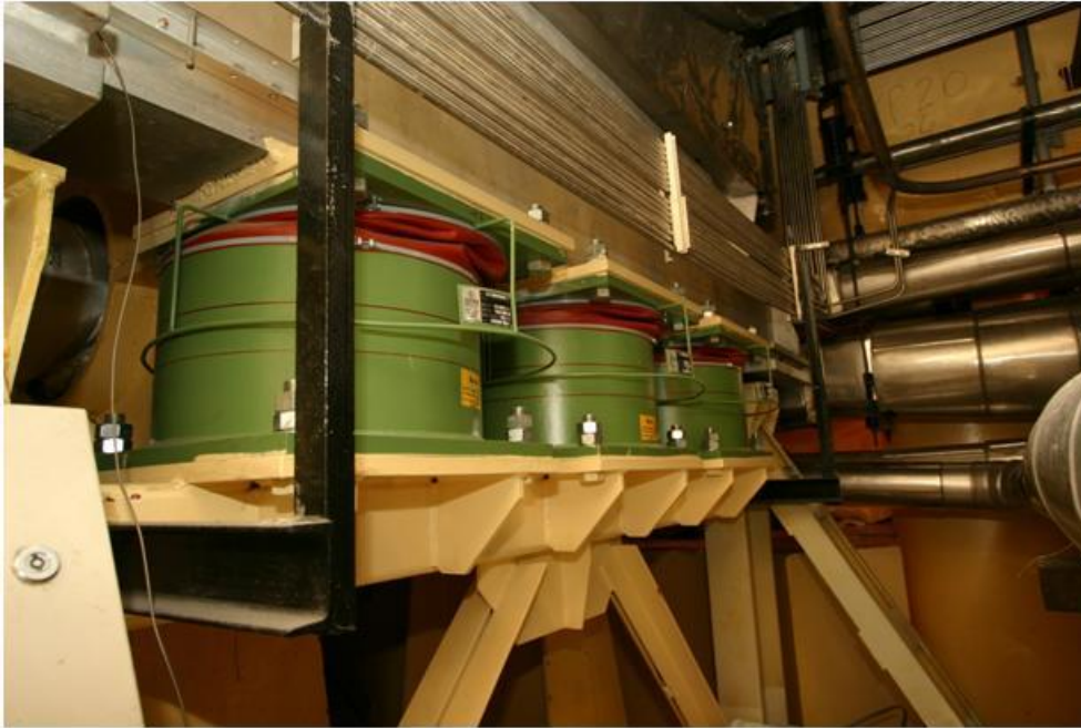
Figure 1-8: Reinforcement by viscous snubbers
