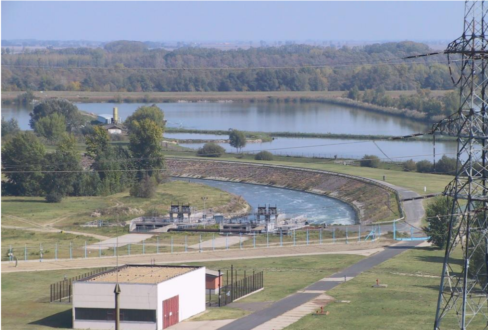
Figure 2-9: Discharge water canal and the fishing lakes
