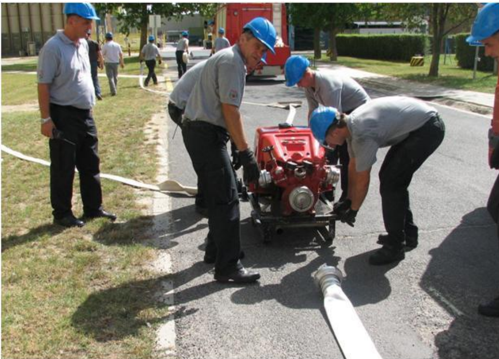
Figure 2-10: Installation of the mobile water intake system
