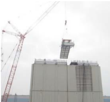
Pictures1: Removal of roof panel
