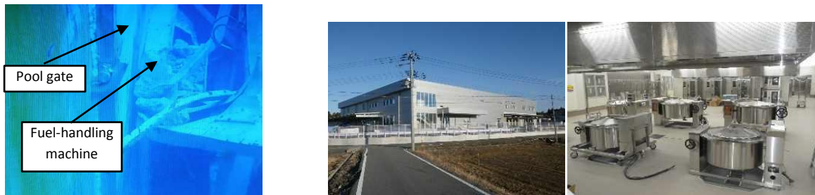
Figure 2: Status of fuel-handling machine in unit 3 SFP and pool gate
