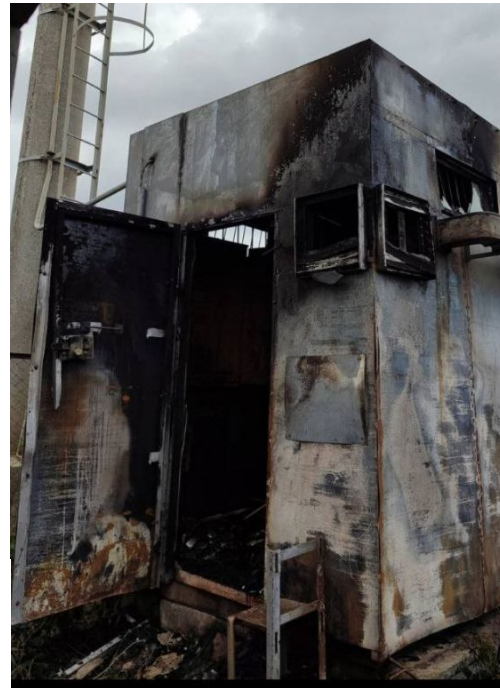
The damaged off-site radiation monitoring station located approximately 16 km to the south-west of the ZNPP. (Photo: ZNPP)
