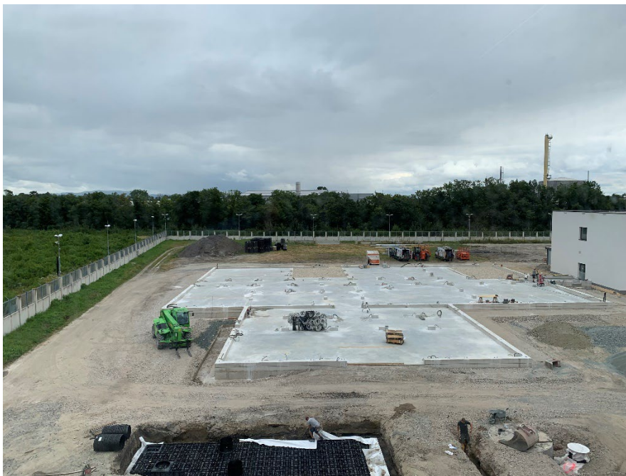
FIG. B.4. Completed greenhouses foundation, July 2024. (Source: IAEA)
