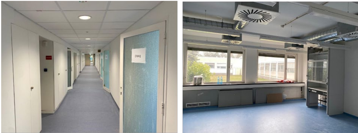
FIG. B.3. Dosimetry Laboratory refurbishment works, March 2024. (Source: IAEA)
