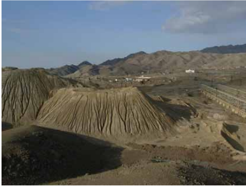
FIG. 4. A tailings pile and acid leach facility at an abandoned site in Taboshar, Tajikistan (note the village and school in the distance).
