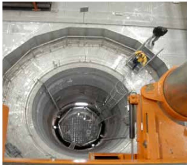
FIG. 6. Inspectors observing the design features of an empty reactor core.
