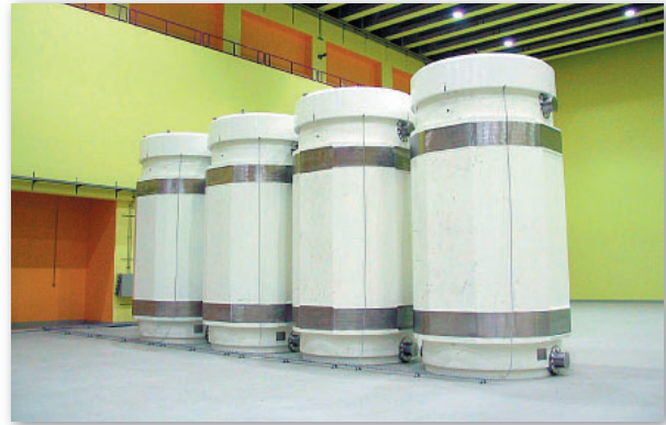
FIG. 2. Interim storage and transport casks at ZWILAG, in Switzerland.
