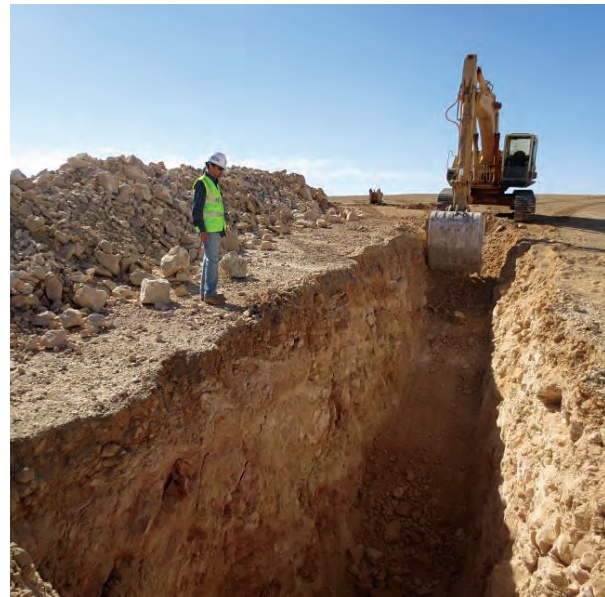
FIG. 1. Excavating an evaluation trench at a uranium deposit in central Jordan.
