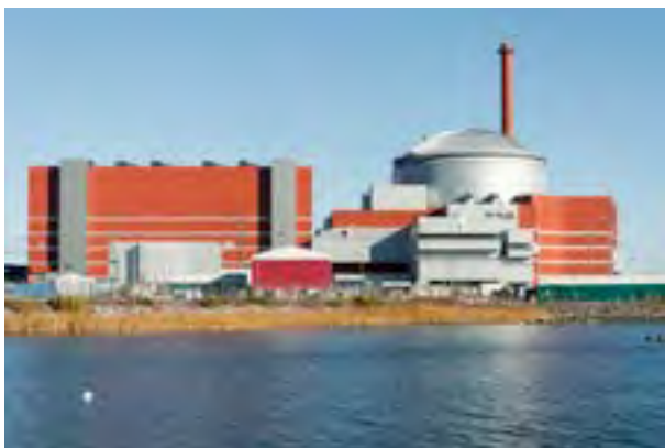
FIGURE 5. Olkiluoto NPP unit 3. Source: TVO.
