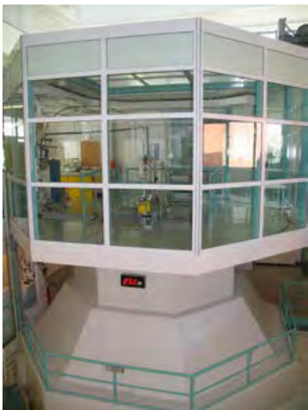
FIGURE 2. FiR 1 research reactor.
