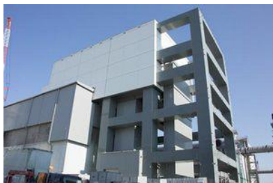
Equipment for fuel removal
