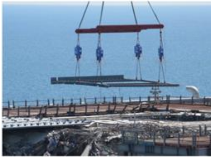
Installing shields on the operating floor
