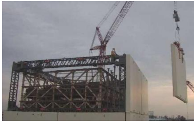
Removal of wall panels
