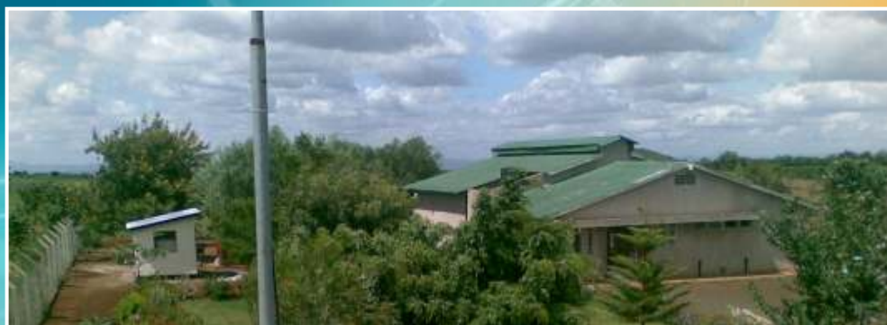
Radioactive waste storage facility in the United Republic of Tanzania.
