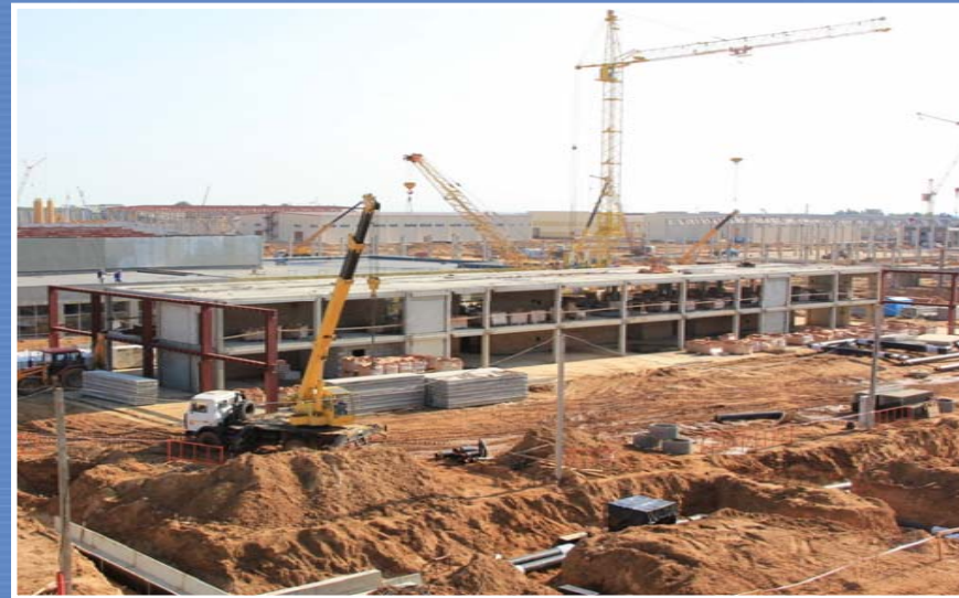
Preparatory work at the Ostrovets site, March 2013
