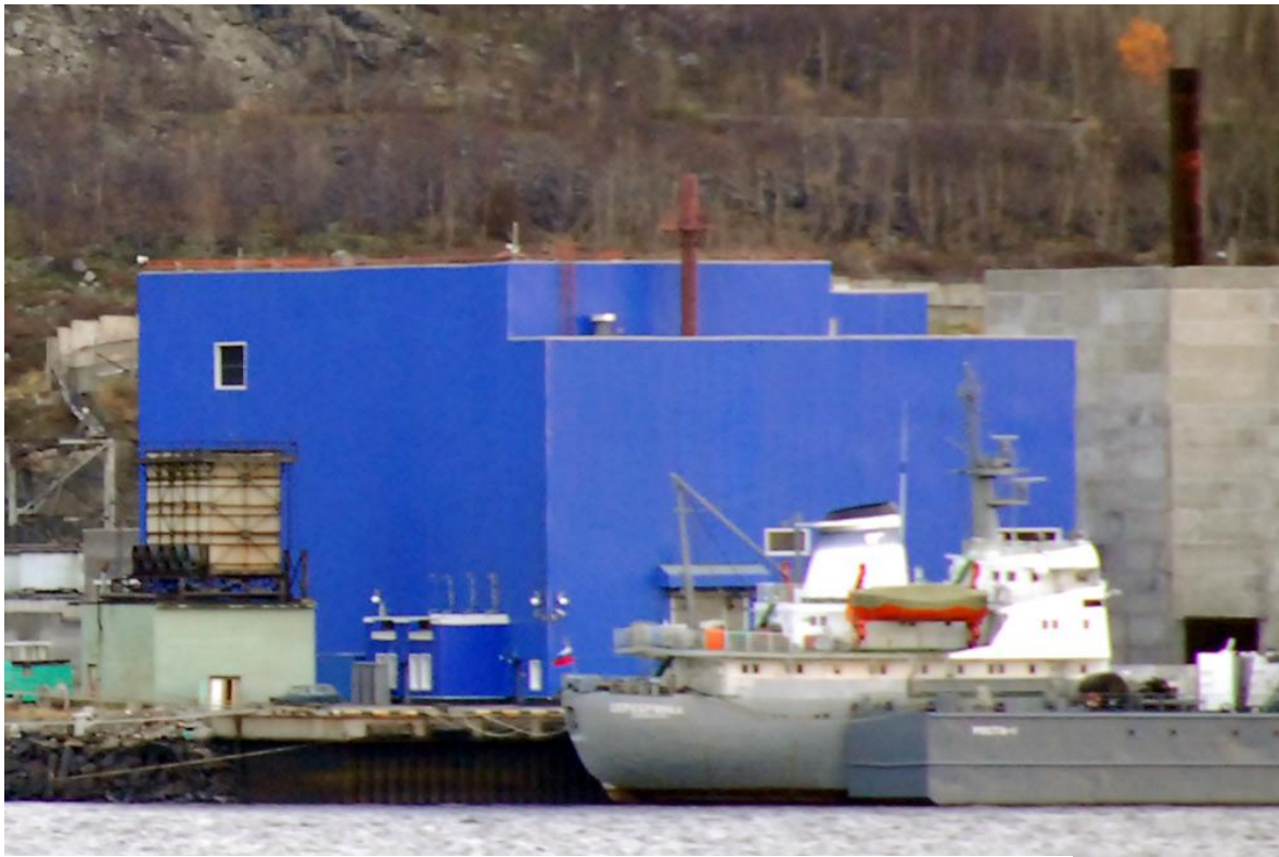
Figure 2. The container-type SNF storage facility at FSUE ATOMFLOT site
