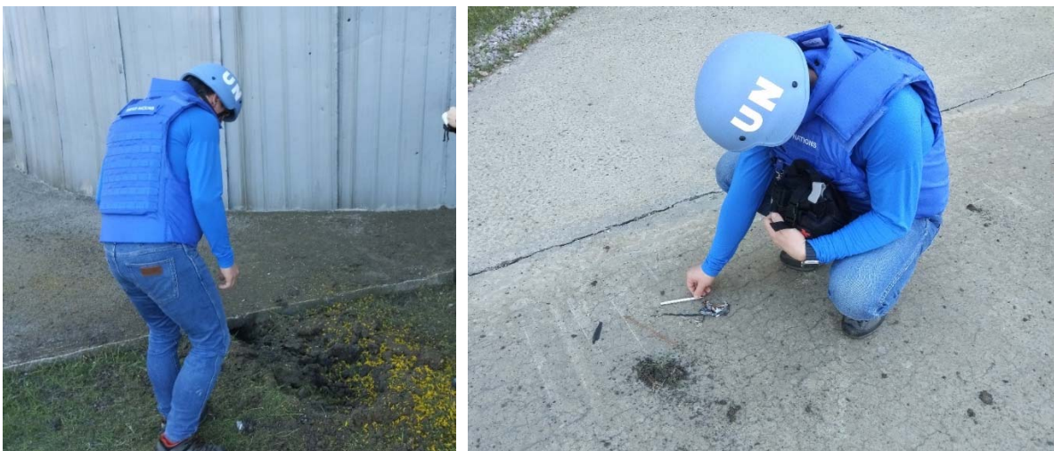
ISAMZ visiting the location of the two connected craters next to the primary make-up water storage tank at the eastern side of the Unit 6 reactor building (left), and observing a piece of foil and part of a rotor blade that appeared to be remnants of the drone (right). (Photo: ZNPP)
