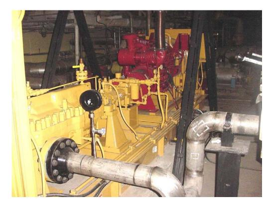
Picture 5. SG Auxliary Make-up Motor Pump
