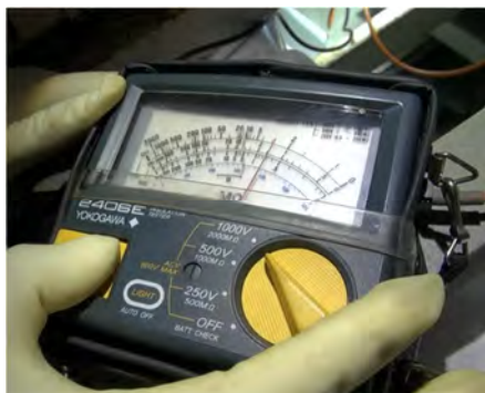
2.8 MΩ between R and S phases
