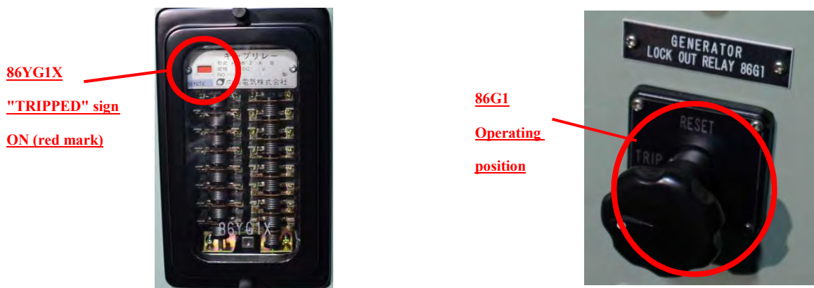
Figure 2.20 Main Generator Lockout Relay
