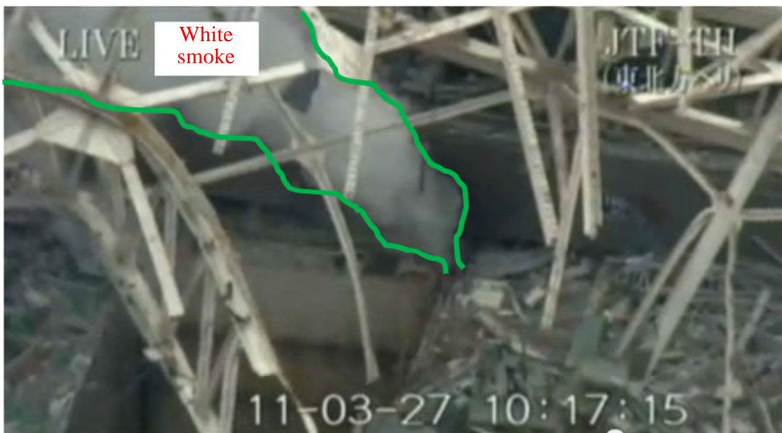
Figure 6.4 White Smoke rising from the Reactor Building of Unit 3 (site 2)
