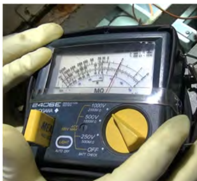
1.9 MΩ between S and T phases
