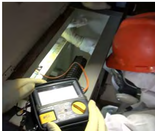
View of measuring an insulating resistance
