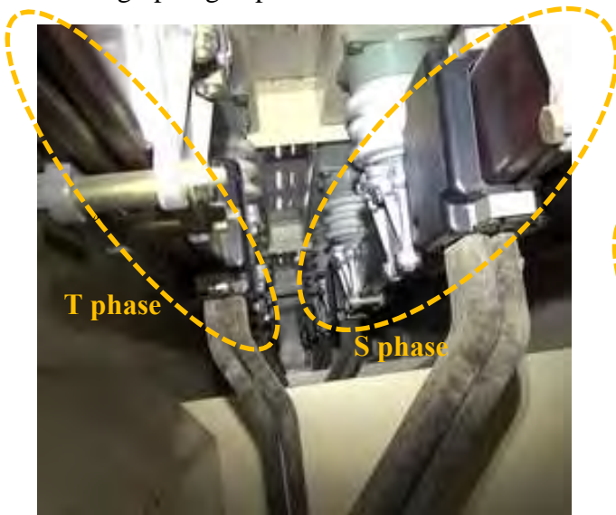
Figure 2.8 Buses and Bus-supporting Insulators inside M/C1C
