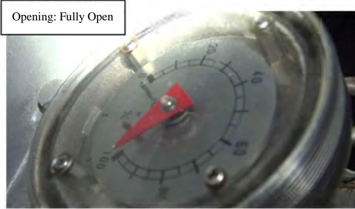
<IC system "A" (2A) opening meter>
