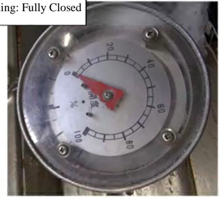
<IC system "B" (2B) opening meter>
