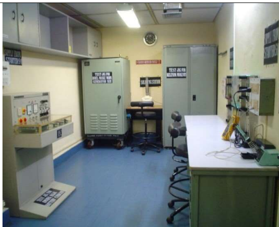
Electrical Card Testing Shop
