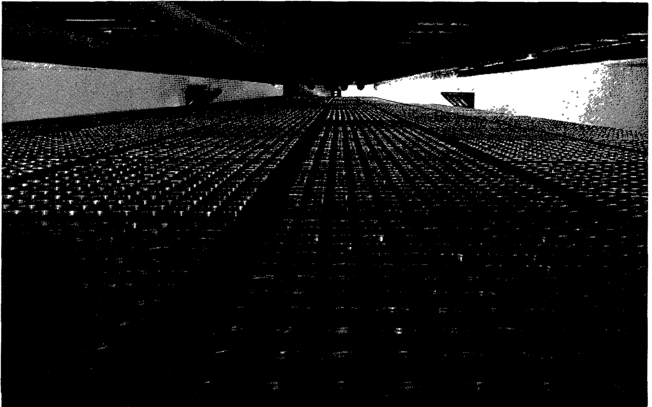
Figure 3a. The vault for dry storage of spent fuel from the gas-cooled reactor at Wylfa, England.
