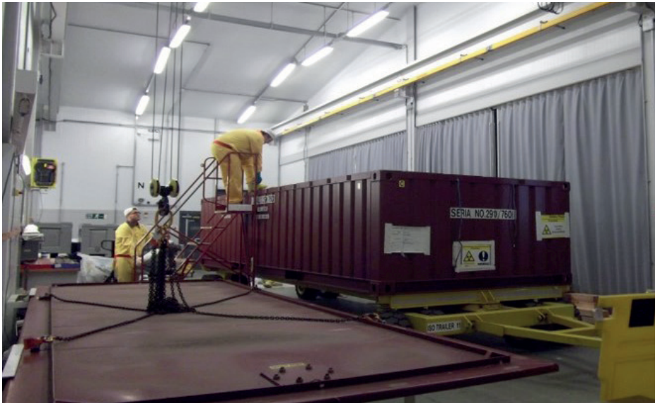
Workers erect a container for receiving wastes generated during decommissioning.
