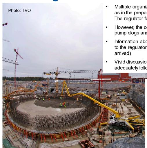
Multiple organizations participated in specifying and testing the concrete mixture, as well as in the preparation and conducting the concreting of the reactor base slab during 2005. The regulator followed the process carefully.
