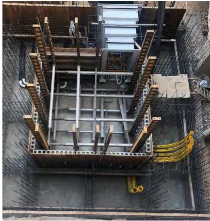
FIG. 6. Wooden frame inside the armor previous the concrete cast
