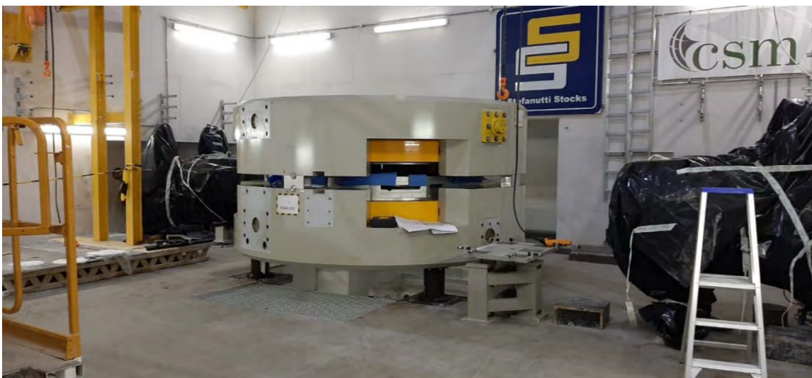
FIG. 5: The C70 cyclotron installed in its final position
