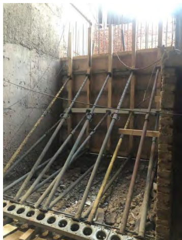
FIG. 10. Shoring system to extern vault wall
