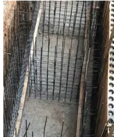
FIG. 7. Double wooden frame inside the armor
