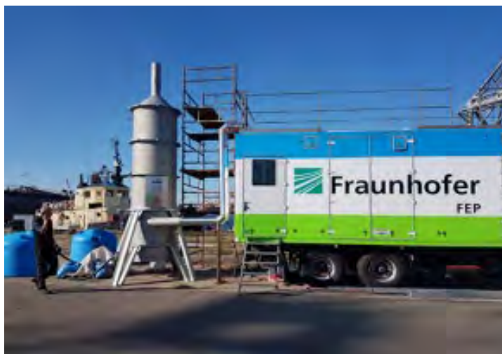
Figure 1: Test of treating the exhaust gases from the diesel engine in a marine tug in Riga harbour using a mobile accelerator from the Fraunhofer FEP Laboratory in Dresden, Germany (courtesy, HERTIS Collaboration)
