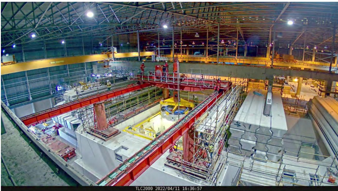
FIG. 4: Rigging of the magnet yokes into the centre vault.
