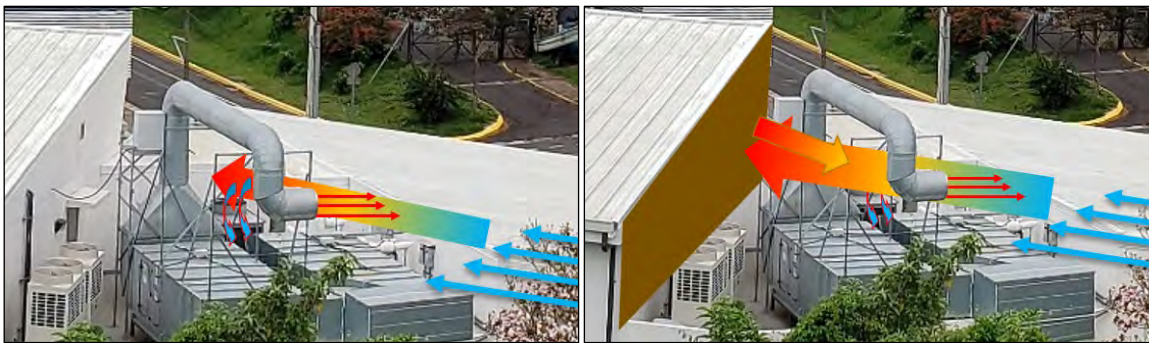
FIG. 2. Wind direction incidence over the inlet/outlet of the HVAC system that generates recirculation. Direct recirculation (left), indirect recirculation (right).
