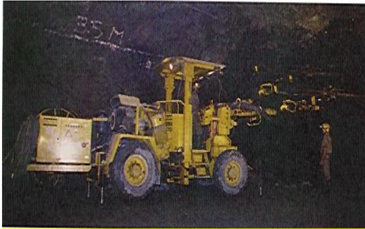
Drilling Operation in Mines (Hydraulic Jumbo Drill)
