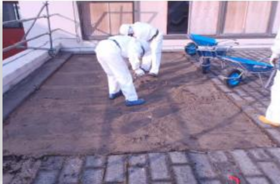
Removal of concrete on admin. building
