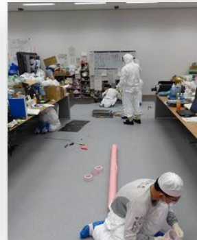
Replacement of floor tiles
