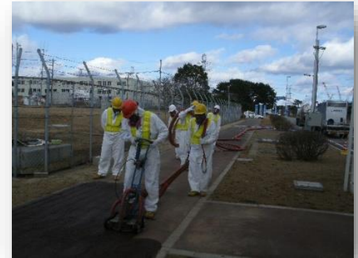
Ultra high pressure water peeling
