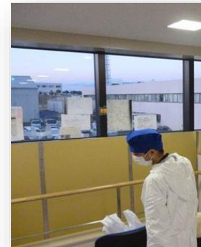
Lead board to shield glass windows
