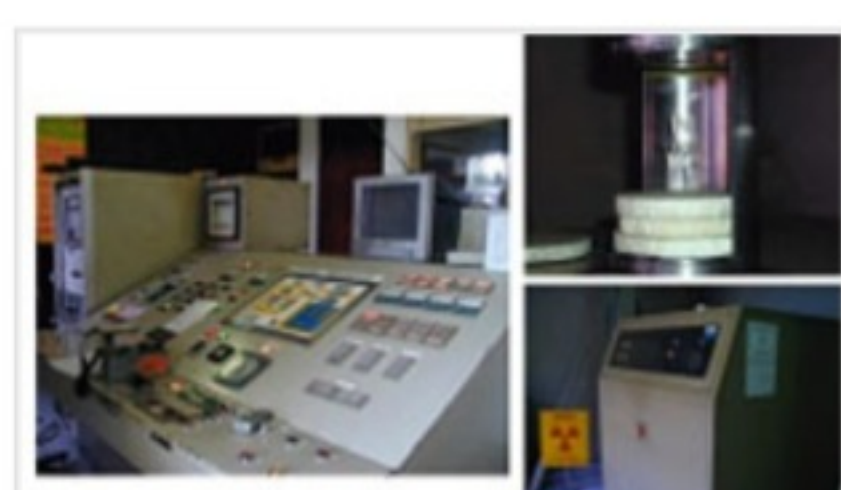
Fig 2. Gamma irradiator facility at CIRA, BATAN
