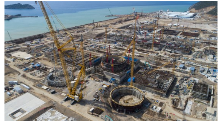
Construction site of the Akkuyu Nuclear Power Plant in Turkey
