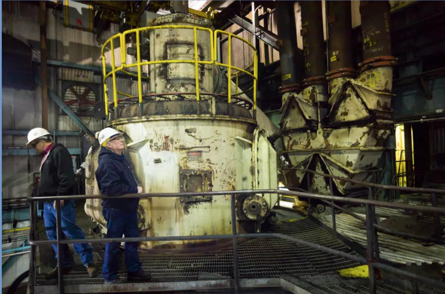
Naughton Power Plant, Wyoming ( wyofile.com )
