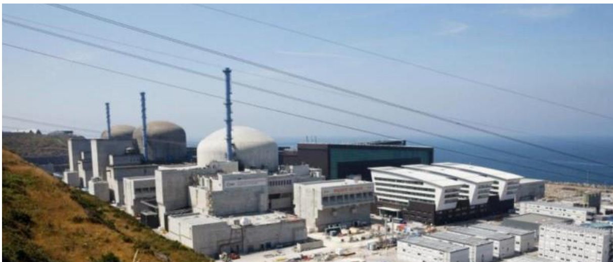
Figure 1: Flamanville 1,2 (1300 MW) and the new Flamanville 3 (EPR 1600MW)
