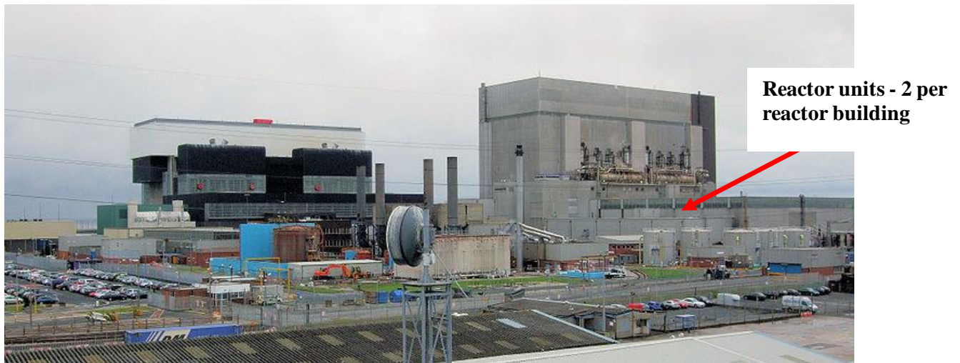
Figure 3A: Heysham 1 (2 x 600 MWe) and Heysham 2 (2 x 615 MWe) Nuclear Power Station, Lancashire, UK – Advanced Gas Reactors. Diagram Source: eDF
