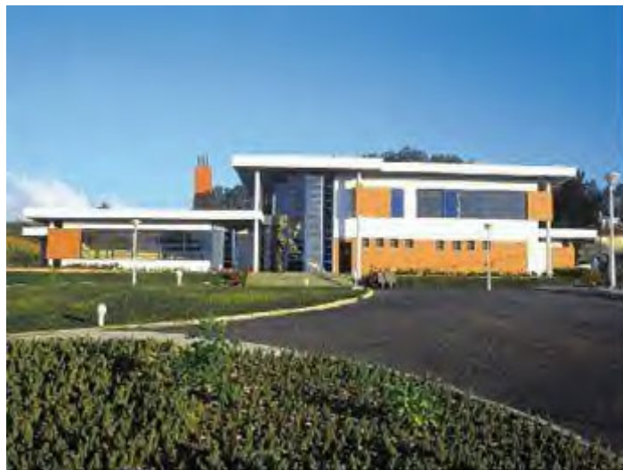
FIG. 5.6. Purpose built Medfly production facility in Madeira, Portugal. (Source: Madeira-Med Web site, 2001)
