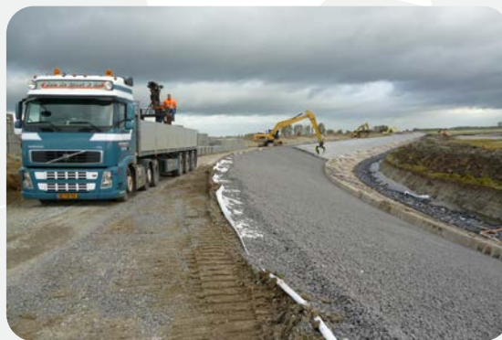
Slag applied in dyke construction Courtesy: Project Organisation Water Safety (NL)
