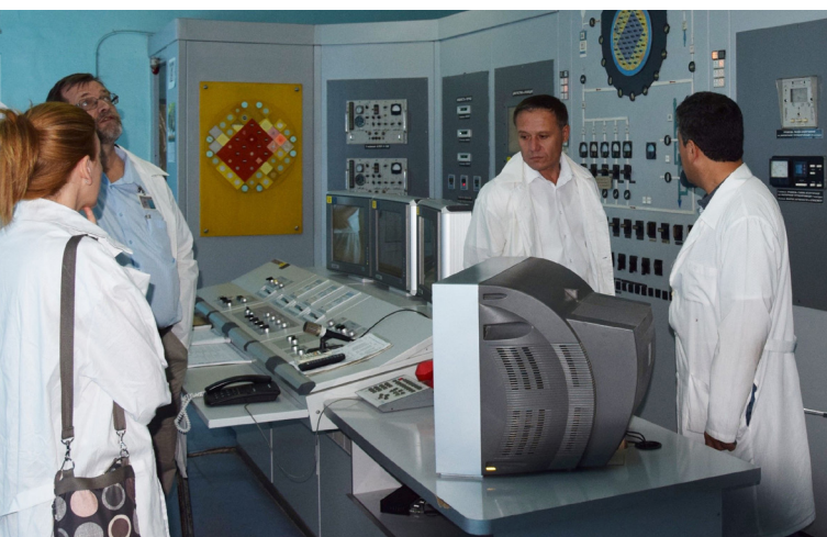
In 2018, the IAEA supported Uzbekistan through an Operational and Maintenance Assessment for Research Reactors (OMARR) peer review mission to optimise operational practices at the WWR-SM reactor. (Photo: Institute of Nuclear Physics)
