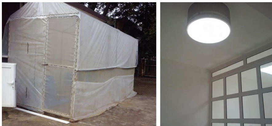
Fig. 10.6 Alternative sources of natural light that can be potentially used for micropropagation. Left image: Shed, lined up with plastic and netcloth, which can be rolled up depending on heat accumulation. Right image: Solatube directs diffused light into the room, without heating the room
