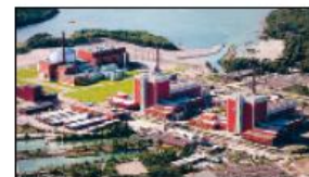
OLKILUOTO, EURAJOKI Owner: Teollisuuden Voima Oyj Reactor units 1&2: EWR 2 x 880 MWe (net) Operation started: 1979, 1982 Production: 14.2 TWh (2010) Load factor: 93.5 per cent (2010) Under construction Olkiluoto 3: EPR (PWR) 1600 MWe Planned: Olkiluoto 4
