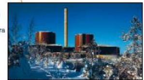
HÄSTHOLMEN, LOVIISA Owner: Fortum Reactor units 1&2: PWR 2 x 488 MWe Operation started: 1977, 1981 Production: 7.7 TWh (2010) Load factor: 91.1 per cent (2010)
