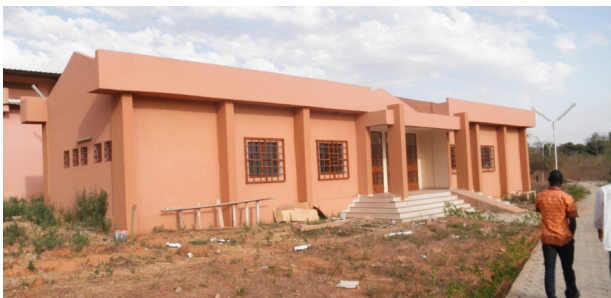
Burkina Faso hosts the largest insect rearing facility in West Africa, applying a nuclear technique to suppress the tsetse fly. (Photo: IAEA)
