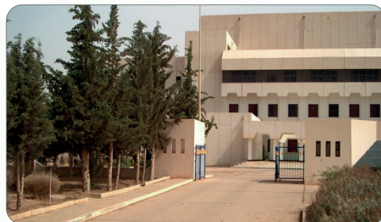
Es-Salam research reactor building
